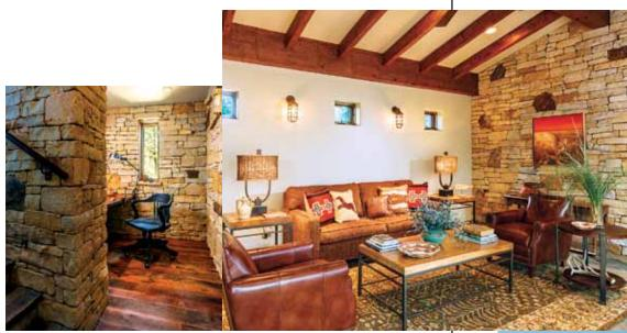
THE SUN Tudor oriented the structure five degrees east of south and staggered its twin stone stacks to create a thermal mass. The sandstone captures the sun's heat during the day and radiates it back when the air grows cool at night. The stone terraces serve the same purpose.
